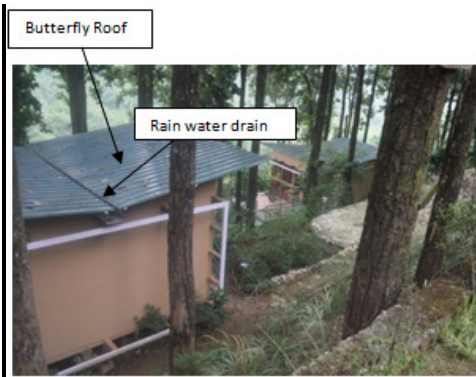
Fig 19: view of Butterfly Roofs
