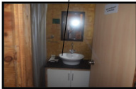
Fig. 17. View of toilet.
